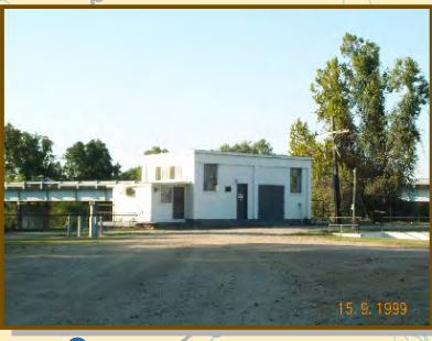
● Plant No. 1 @ Bay City
