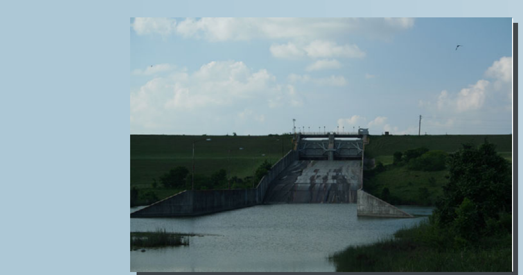
Photo 12. Walter E. Long dam operated by the City of Austin near FM973, Decker Creek flows into Gilleland Creek.
