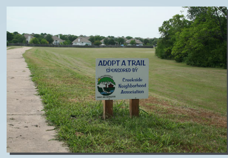
Photo 6. Embankment of Creekside Park flood detention pond in Pflugerville.
