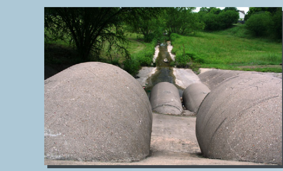
Photo 5. Staggered overflow tubes in embankment of flood detention pond in Moose Park in Pflugerville.
