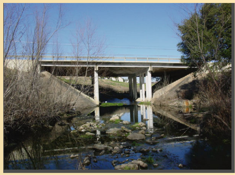
Photo 14. Looking upstream at the FM 1431 Bridge.
