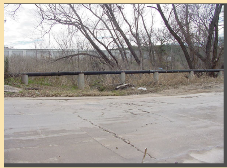
Photo 36. Commerce Street, elevated wastewater line on downstream side of street.
